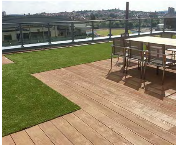
Decking & Artificial Turf
